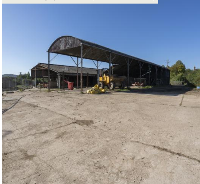
Ground Photograph of the site (taken from the north)
