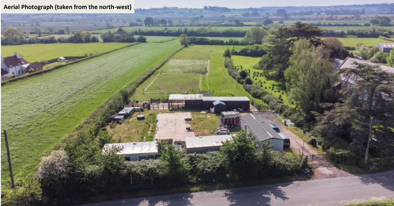
Aerial Photograph (taken from the north)
