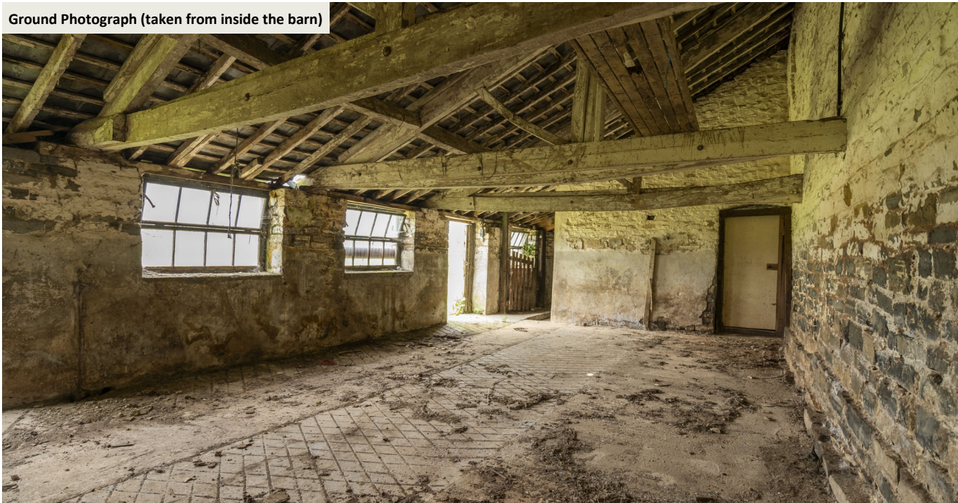
Ground Photograph (taken from inside the barn)
