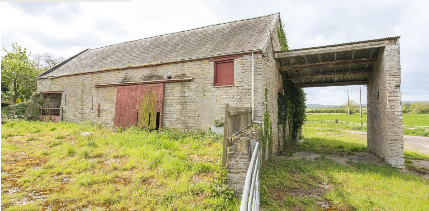
Ground Photograph (taken from the north)
