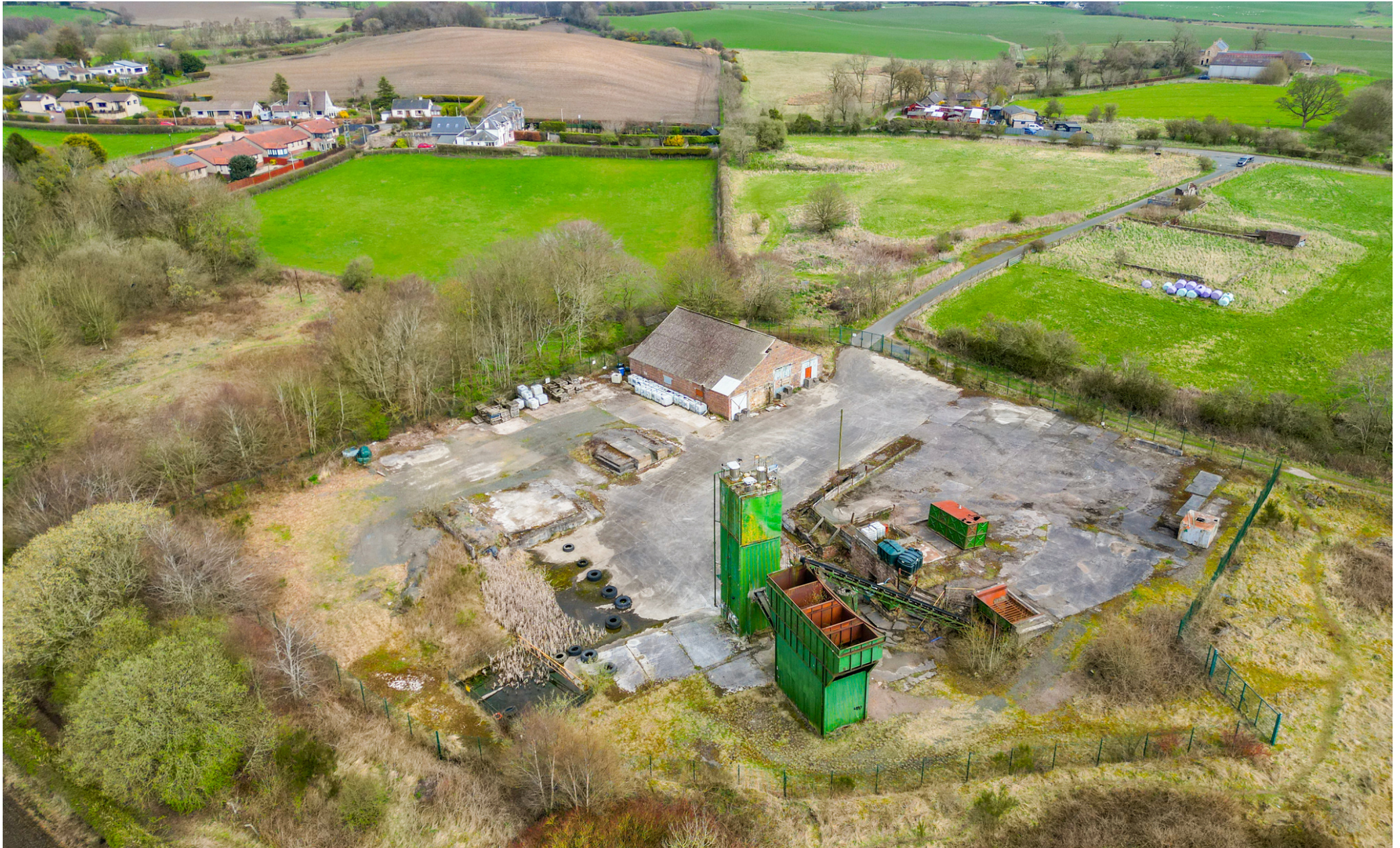
Aerial photo of the site looking northeast
