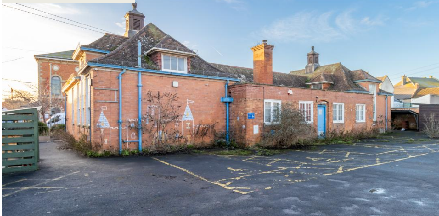
Ground photograph (taken from the north)
