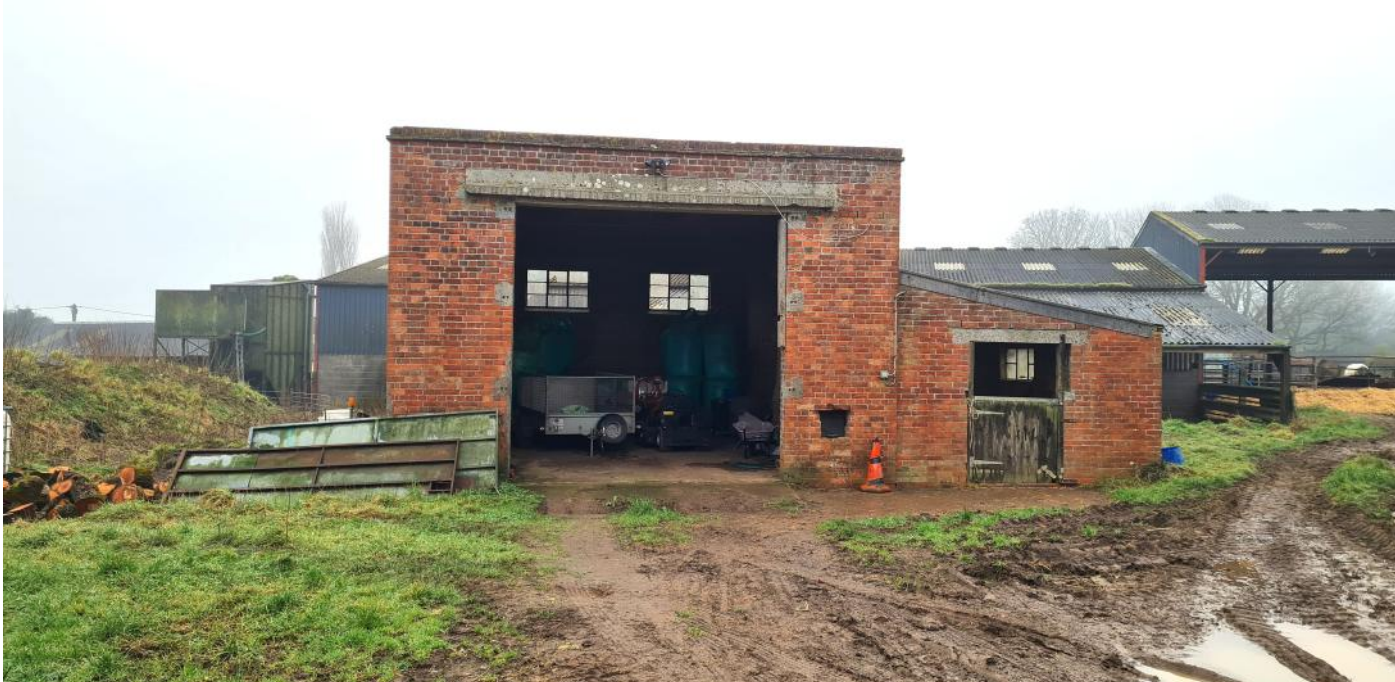
Ground photograph (taken from the north)
