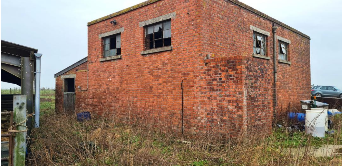
Ground photograph (taken from the north)
