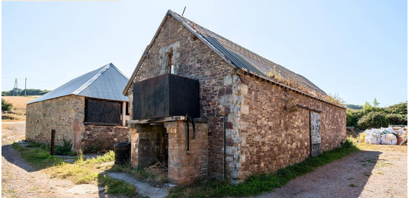
Ground photograph of the Store
