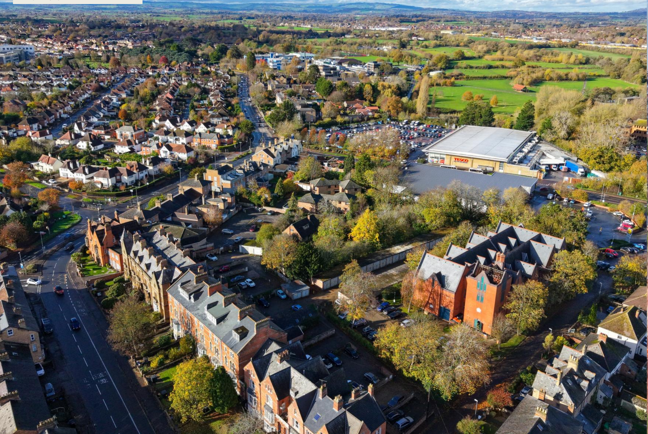
Aerial photograph taken from the south-east
