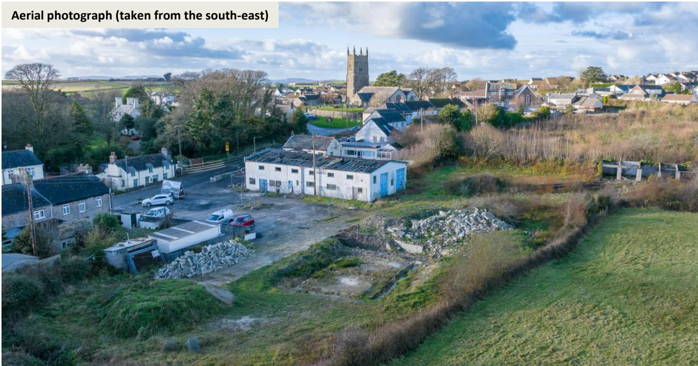
Aerial photograph (taken from the north)
